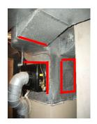
Place on ducts to eliminate the hot/cold/hot boom, on all seams to seal up your HVAC and stop wasting dollars in lost a/c and heat.
